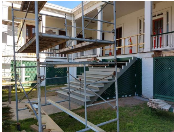
Beauvoir's back steps are finally getting replaced and are near completion.
